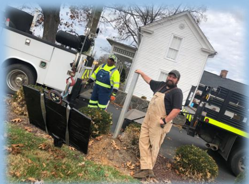
Foundation for the Boarding House Sign.
