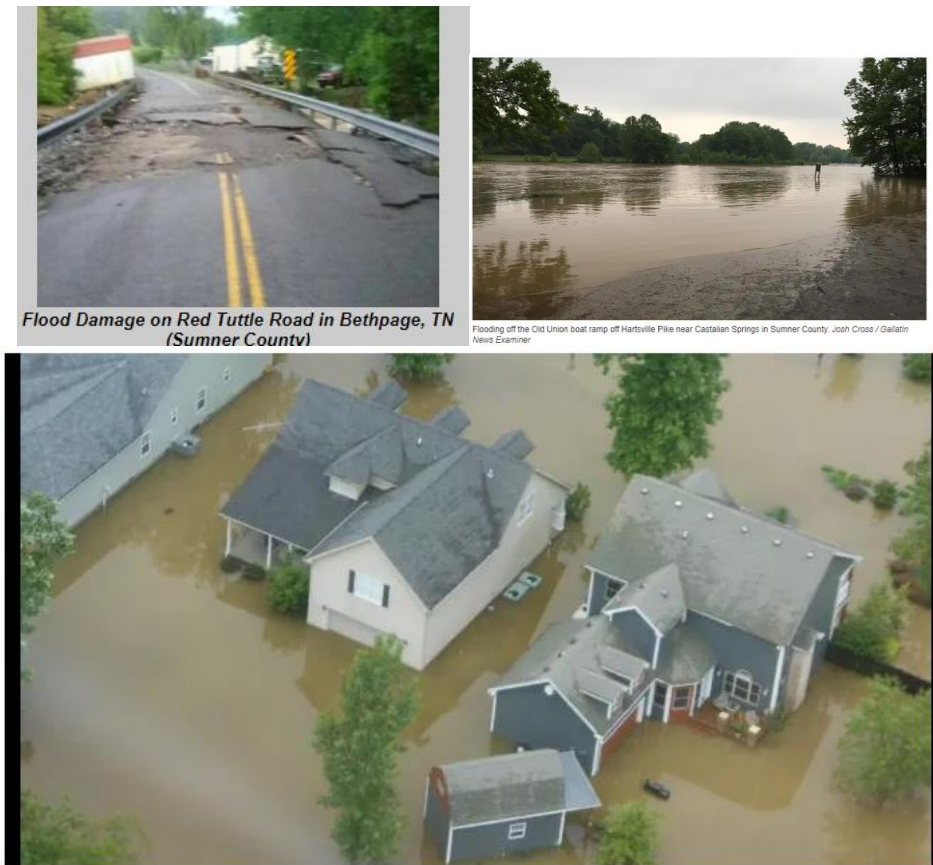
Figure 13: May 11, 2016 Floods damage and depths (The Tennessean)
